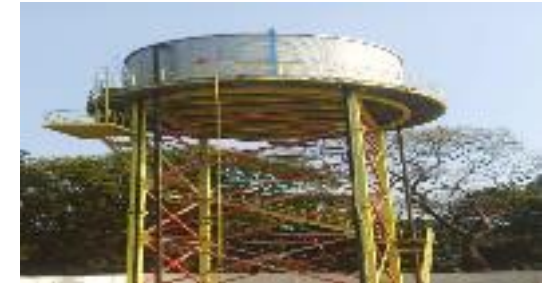
Water Tank, Uttar Pradesh
